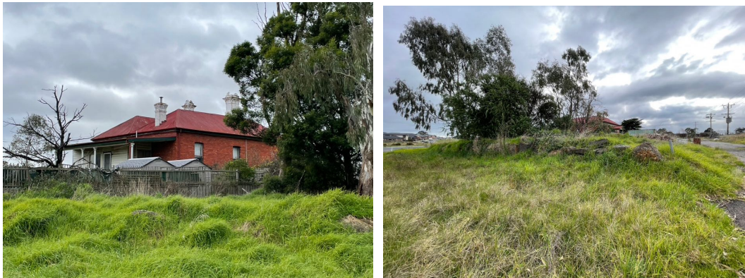
Figure 6: South and west elevations of the house and the dry stone retaining wall along the north boundary of Station Lane (Source: David Helms 2023).
