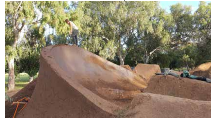
City Dirt Crew constructing berm, with drainage visible at base
