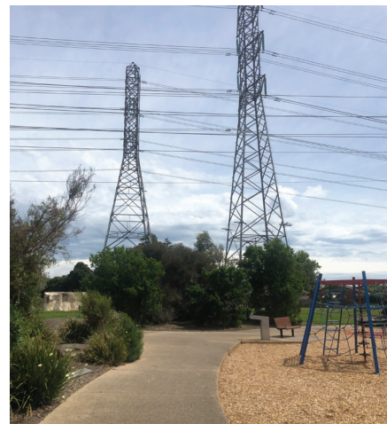
Figure 17. Electricity Transmission Corridor & Towers
