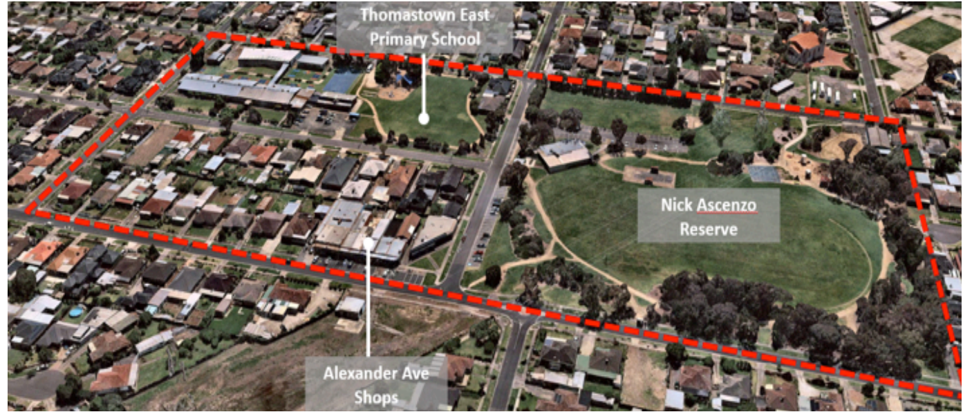
Figure 2. Alexander Avenue Precinct
