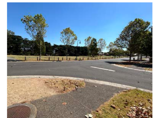
D Lack of pedestrian crossing facilities
