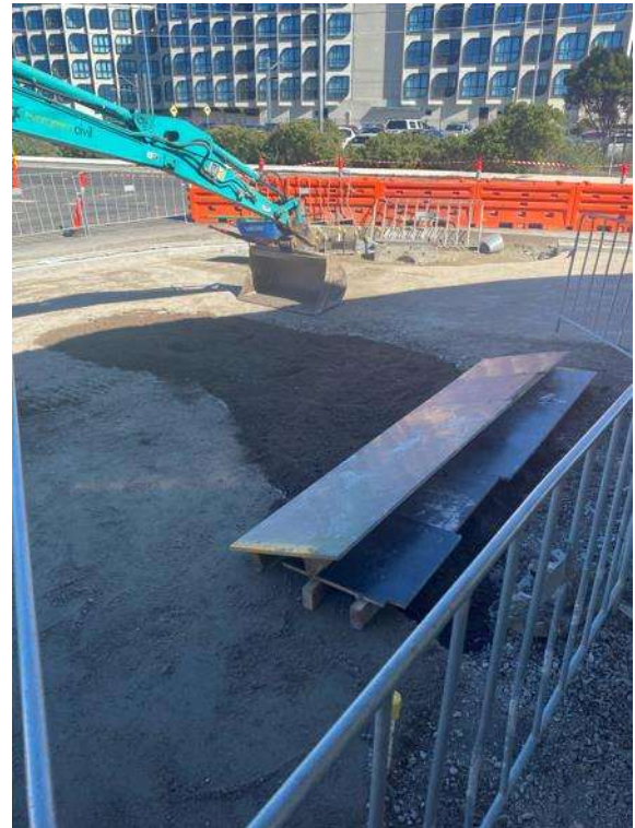
Excavation works on the corner of Station Street and The Boulevard
