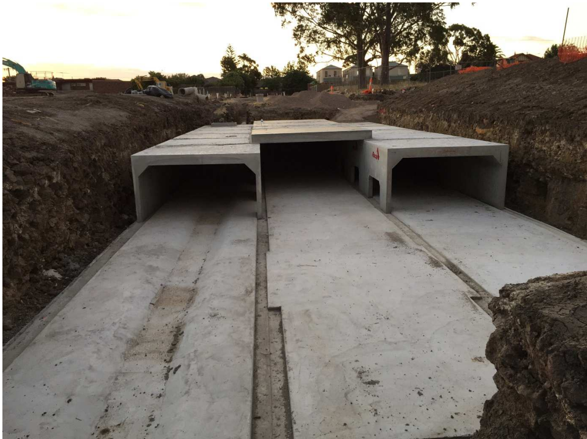
Figure 3– Photo of an underground detention system during construction
