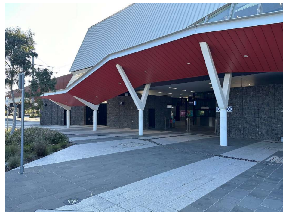
Figure 19: Hawkstowe Rail Station
