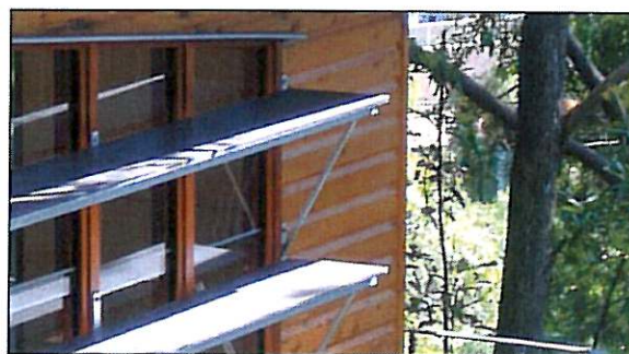
Cross ventilation and sun shading reduce the energy consumption of buildings.
