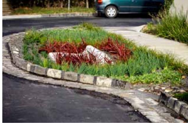
**Figure B-2: Bioretention Basin** Source: Melbourne Water.
