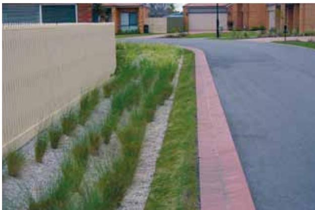
**Figure B-1: Bioretention Swale**
