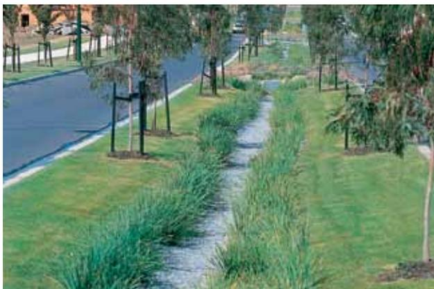
**Figure B-3: Vegetated Swale** Source: Melbourne Water.
