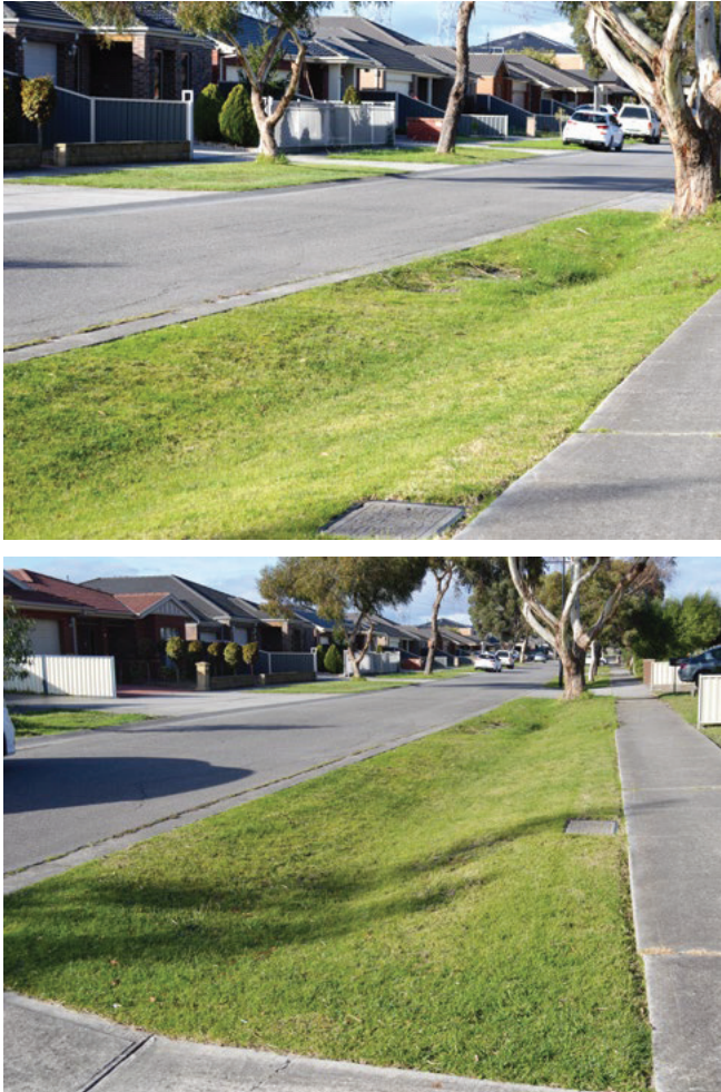
Figure 4 Examples of drainage swale/channels.
