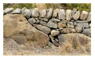
**Figure 15** Stone Size – Cyclopean common-sized stones complete the upper portion of the wall.
