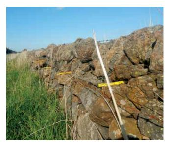
Figure 29 Throughstone Placement - Projecting. Yellow pegs have been placed to highlight each projecting
