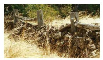
Figure 6 Structural Components – Stone and Timber Post and Rail. The wooden rails are badly weathered. Note the lower mortice in the post on the far right, suggesting possibly, an earlier post and rail fence.
