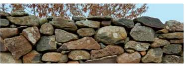
Figure 24 Coping Pattern - None. Figure shows wall levelled to height with small stones but not described as cope stones.
