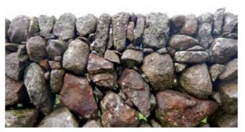
Figure 8 Construction Style – Single wall.
