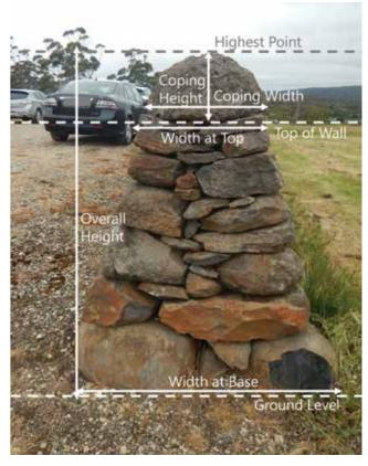
Figure 35 Cross-section of a dry stone wall.
