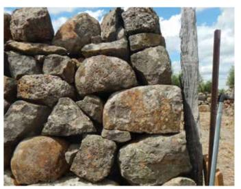
**Figure 16** Stone Size – Oversized. Figure shows a wall end and section of face.
