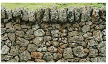
**Figure 14** Stone Size – Common. Stone is of a size which is easily lifted and placed in the wall.
