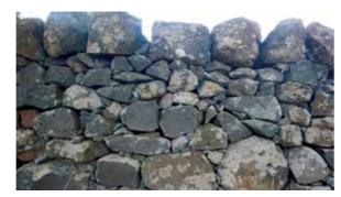
**Figure 11** Stone Type – Basalt. Stone shows a small amount of vesiculation and lichen growth on the natural stone surfaces.
