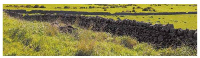
**Figure 31** Subjective Condition – Very Good. Two wall sections in substantially original condition downgraded due to the isolated gaps and missing copestone.
