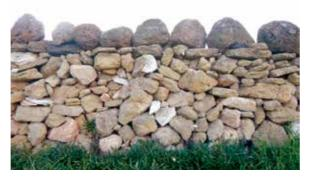
**Figure 13** Stone Type – Limestone. The copestones are vesiculated basalt.
