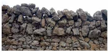
Figure 10 Construction Style - Galloway wall. This example built with highly vesiculated basalt stone. Vesiculated basalt having visible surface holes or cavities in the rock.
