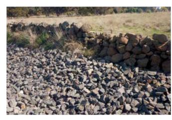
**Figure 34** Subjective Repair Quality – Poor. A rubble wall (right) has been reinstated to join a Galloway style wall (left). The Galloway wall is in fair condition. The stone fill in the foreground is recent and placed in the roadside "gutter."
