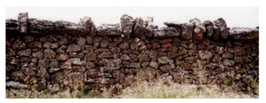
Figure 28 Coping Pattern – Cock and Hen. Multiple uprights and flats are repeated to form the pattern.
