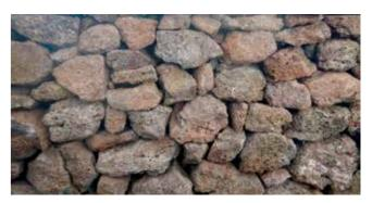
**Figure 23** Stone Surface – Vesicular, with naturally occuring holes.
