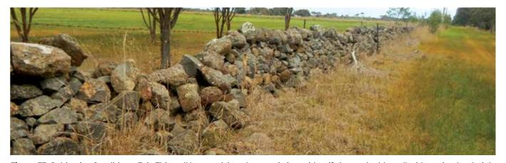
**Figure 33** Subjective Condition – Fair. This wall has surviving characteristics to identify it as a double wall with coping but height is variable due to collapse and slumping. Fallen stone has been crudely returned to the gaps.
