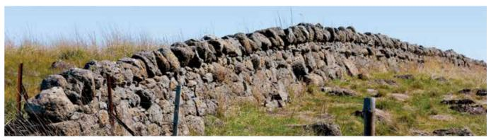
**Figure 30** Subjective Condition – Excellent. A length of wall in original condition for line, height, style with no missing stone. Note the line of projecting throughstones.
