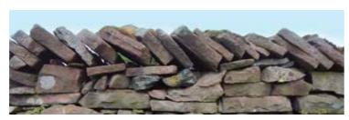
Figure 27 Coping Pattern – Inclined.
