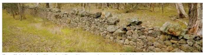
Figure 32 Subjective Condition – Good. The wall has many minor gaps but full-height wall remains.
