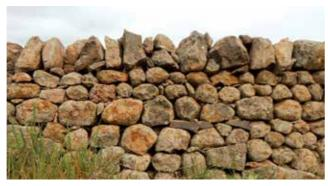
Figure 17 Stone Shape – Rounded.
