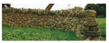
Figure 9 Construction Style - Double wall. The wall end at right, shows the wall's cross-section detail.
