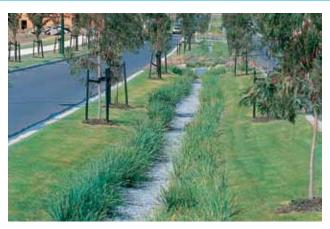
Figure B-3: Vegetated Swale Source: Melbourne Water.
