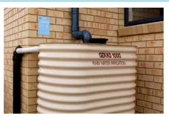
Figure B-8: Rainwater tank Source: Melbourne Water.
