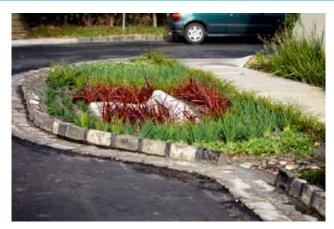
Figure B-2: Bioretention Basin Source: Melbourne Water.
