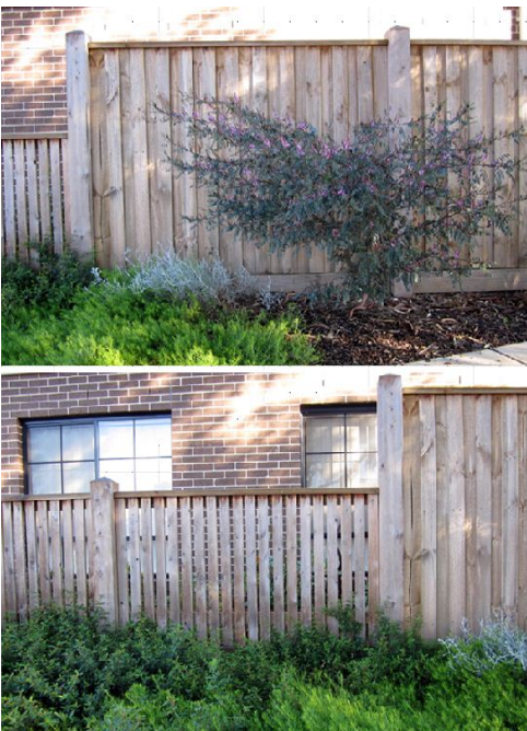
TYPICAL TIMBER PALING AND PICKET FENCE
