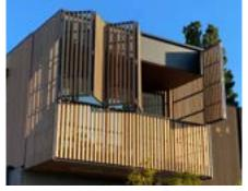
Figure 22 External blinds, louvered or screened shutters provide greater sun control in various seasons.
