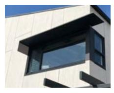
Figure 23 Windows with hoods maximise access to winter sun and minimise the heat of summer sun, especially
