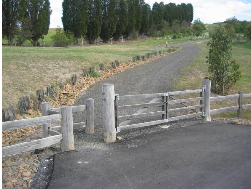
Swamp Gum Gully pedestrian access and maintenance gates (The pedestrian opening needs modification to exclude motor bikes but allow access for prams and wheelchairs)
