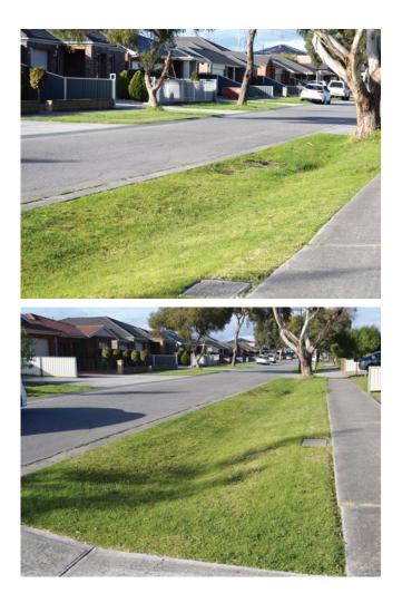
Figure 4 Examples of drainage swale/channels.
