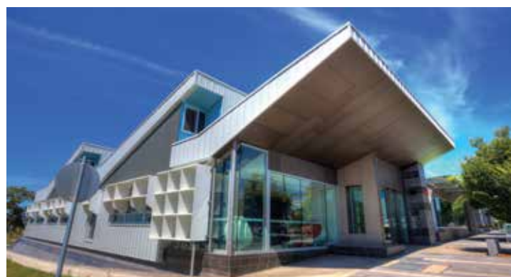
Epping Views Family and Community Centre
