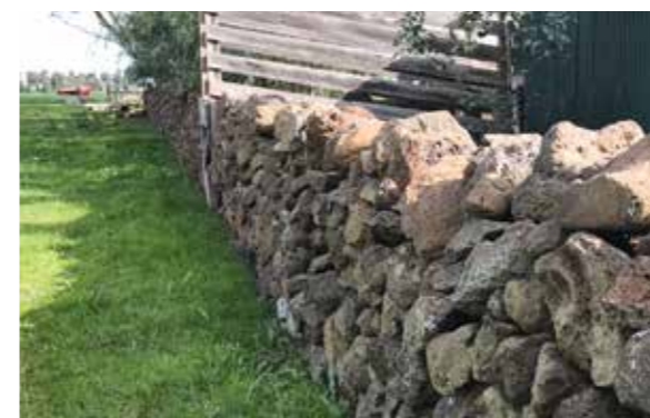
Top left and above: All stone double wall, Cobblebank. Source: City of Melton Below left: All stone double wall, Toolern Vale. Source: City of Melton Right: Source: Shutterstock
